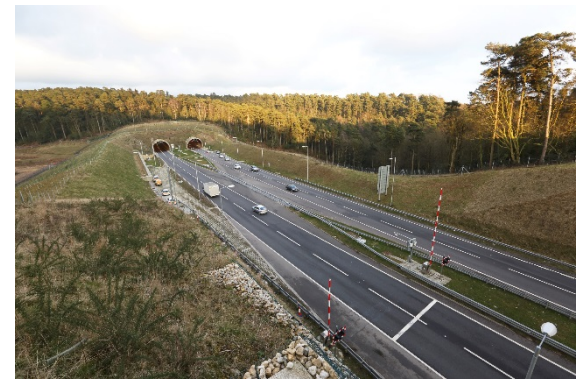
«Hindhead Tunnel 12». Highways Agency. https://www.flickr.com/photos/highwaysagency/ https://flic.kr/p/eHWF1X https://creativecommons.org/licenses/by/2.0/
