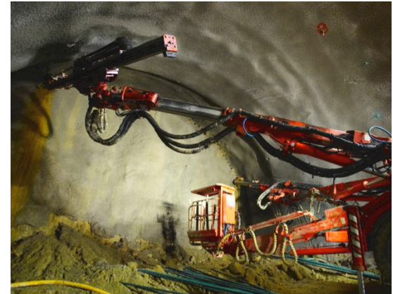
«Tunnel construction». Highways Agency. https://www.flickr.com/photos/highwaysagency . https://flic.kr/p/9TZCmQ . https://creativecommons.org/licenses/by/2.0/ .
