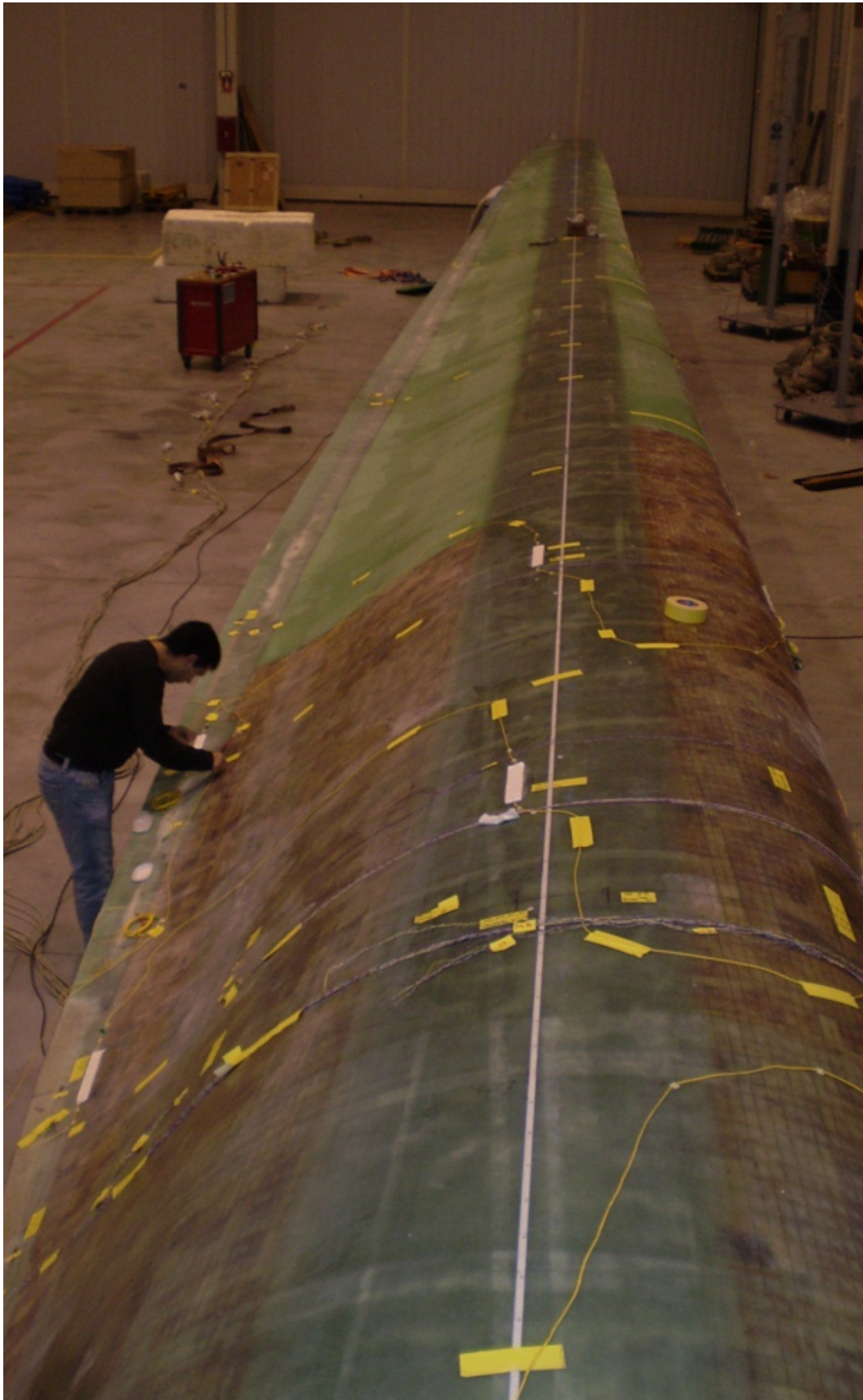
Figure 16. Installation of optical fiber sensors based on diffraction gratings on the blade of a wind turbine. Source: Photonics Engineering Group at the University of Cantabria.
