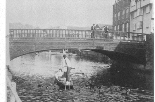
Fig. 1.4. Magdalene Bridge built in 1823 on the site of the ancient Saxon bridge over the Cam. The present cast-iron arches carried, until recently, loads far in excess of those envisaged by the designers. Fortunately, the bridge has now undergone a well-earned restoration.
