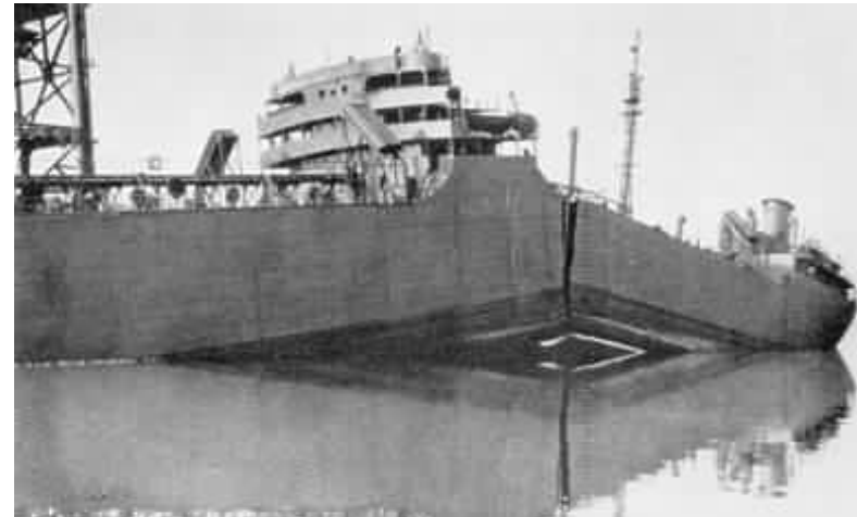
Liberty ship which was broken in two halves along the welds.
