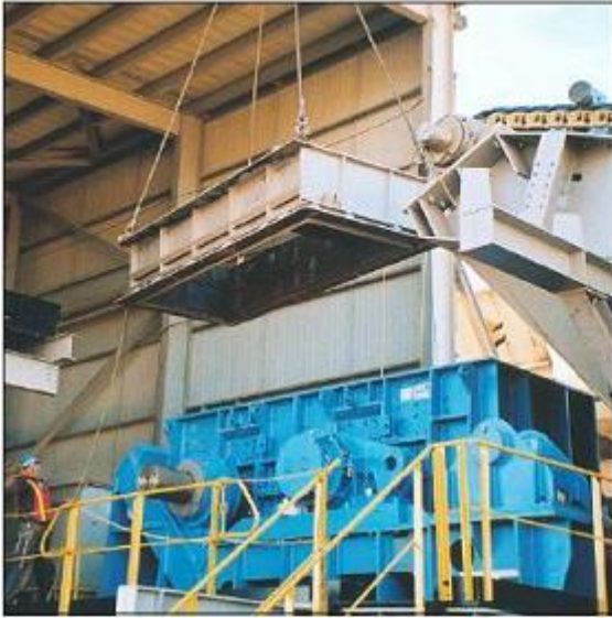
Crushing plant in Canada with double roller crusher SZWB2015 and apron feeder AF 2400 x 14
