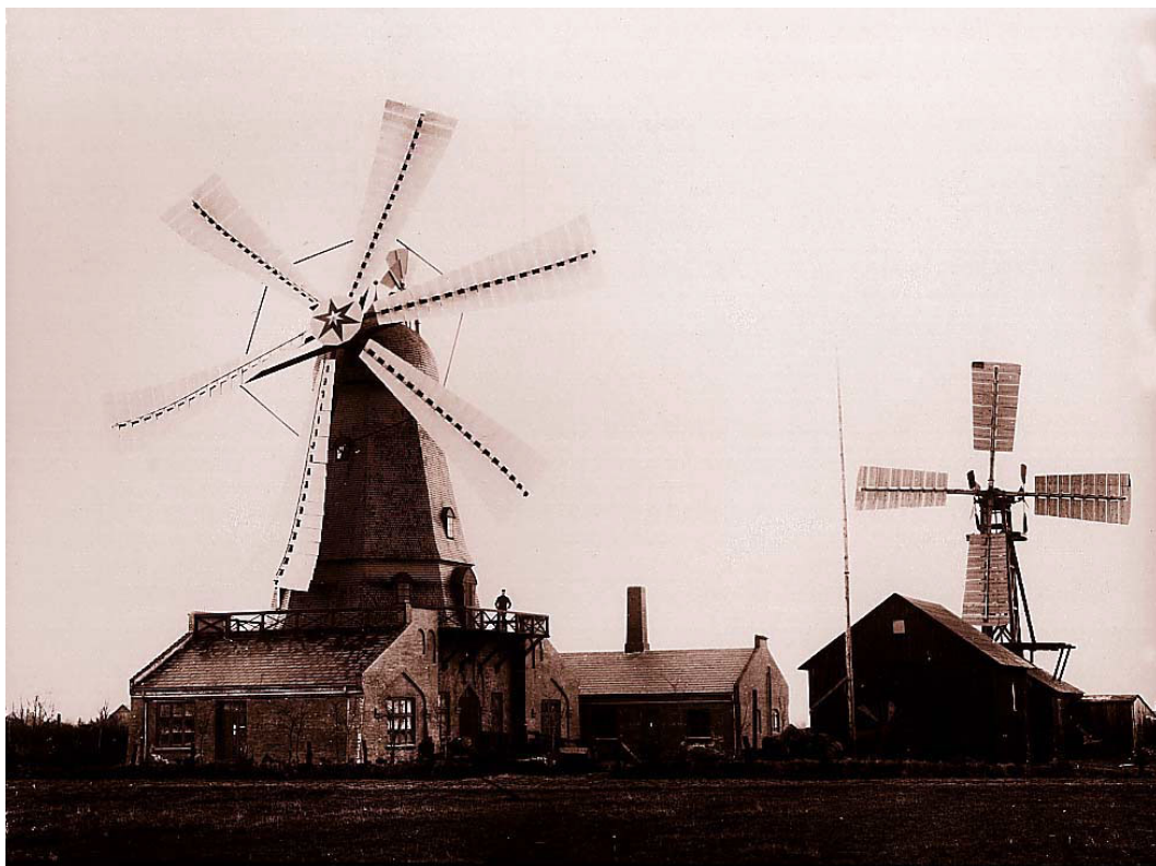
Figure 2. Two test wind turbines by Poul la Cour in the Askov Folk Institute, Askov (Denmark, 1897). Source: http://bit.ly/2mFUIfm . License: Copyright 1997-2003 Danish Wind Industry Association.
