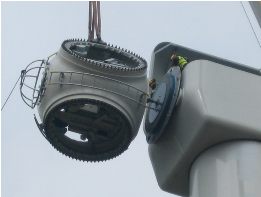
Figure 42. Wind turbine hub being connected to the nacelle. Source: Wikimedia. License: CC-BY-SA 2.0
