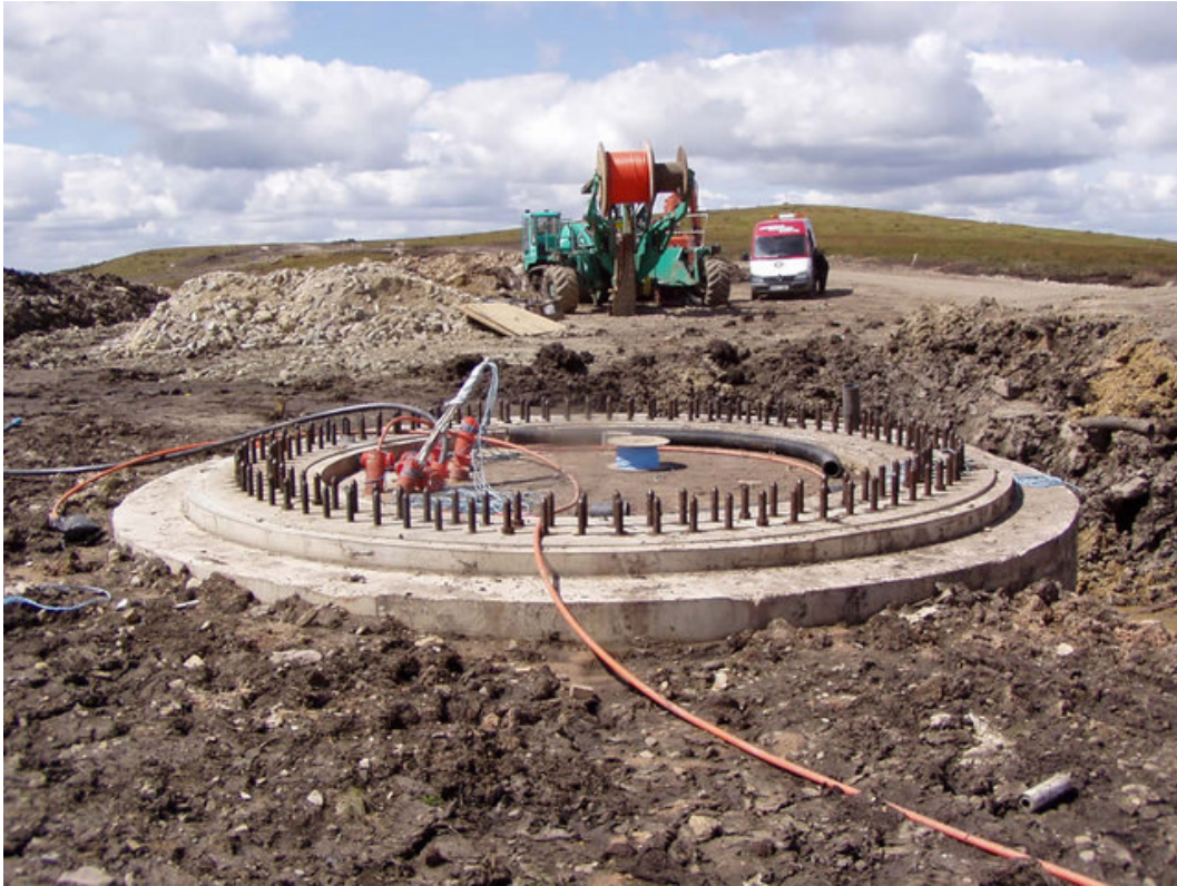
Figure 36. Foundations of an onshore wind turbine. Source: Wikimedia. License: CC BY-SA 2.0. http://bit.ly/2mLQ6nZ
