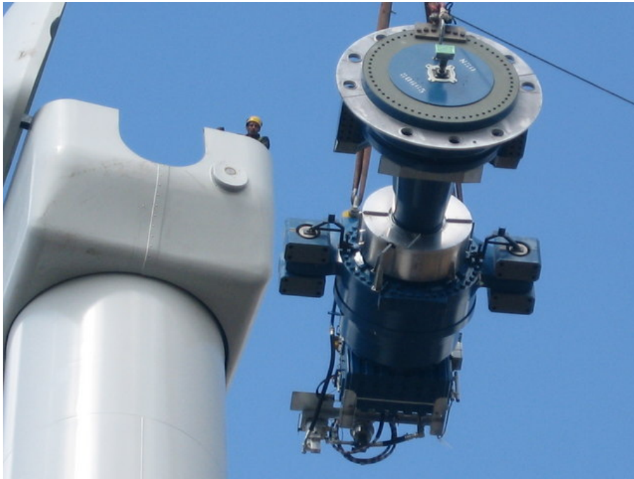
Figure 46. Gear box, rotor shaft and brake in a wind turbine. Source: Wikimedia. License: CC BY-SA 2.0. http://bit.ly/2ERH8Mx
