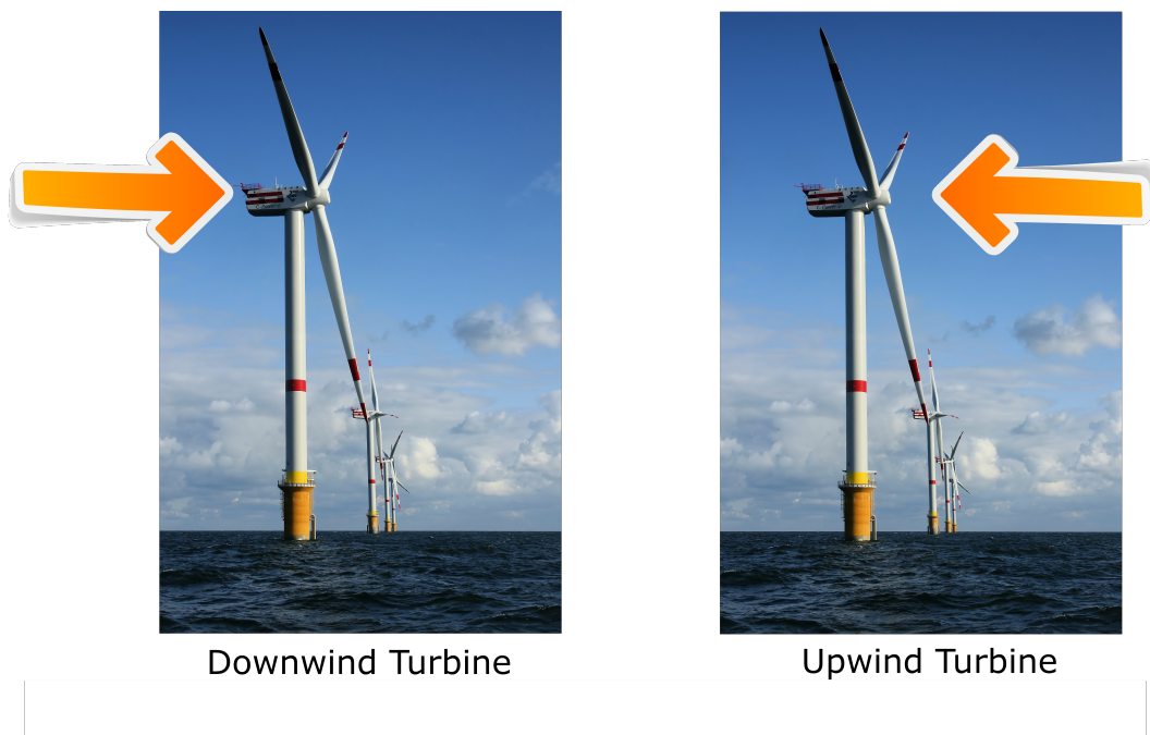
Figure 45. Upwind and downwind turbines. Source: Wikimedia. License: CC BY-SA 4.0 Attribution (© Hans Hillewaert) http://bit.ly/2EPJ0Fp .
