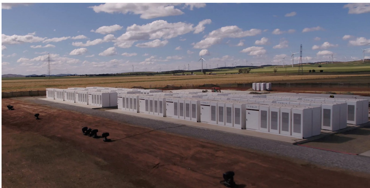
Figure 1.52. Tesla PowerPack Project at Hornsdale (Australia). Source: electrek http://bit.ly/2DJsw0W
