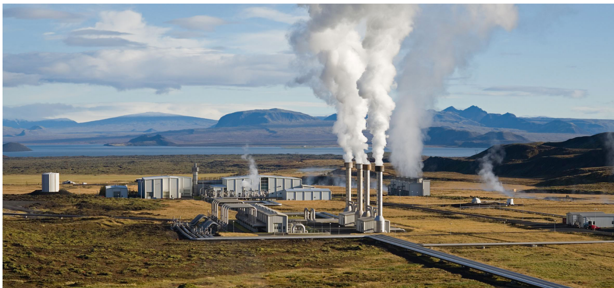
Figure 1.3. Vapour emitted by the geothermal power plant in Nesjavellir (Iceland). License: Public Domain (Gretar Ivarsson). https://bit.ly/2S2N0cL
