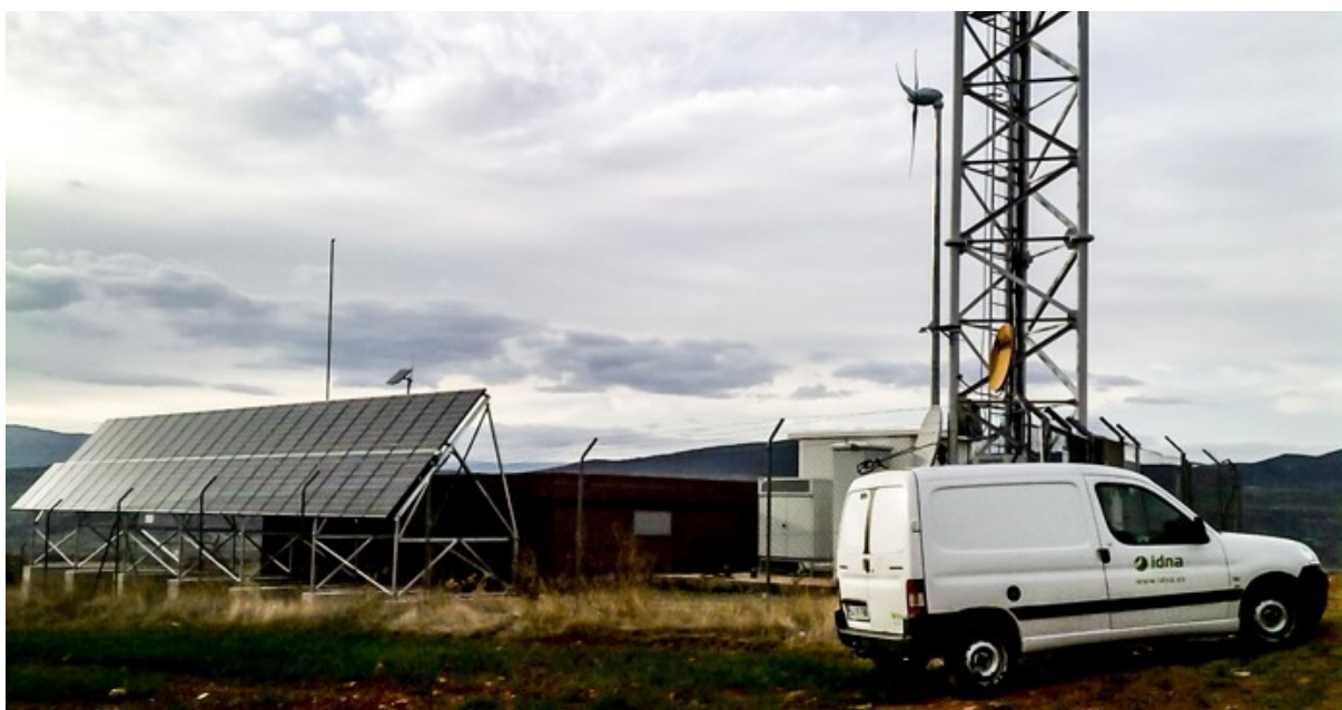
Figure 1.54. Example of a small solar-PV and wind power system associated with a TDT station in Uceda (Guadalajara, Spain). http://bit.ly/2AZw1ya
