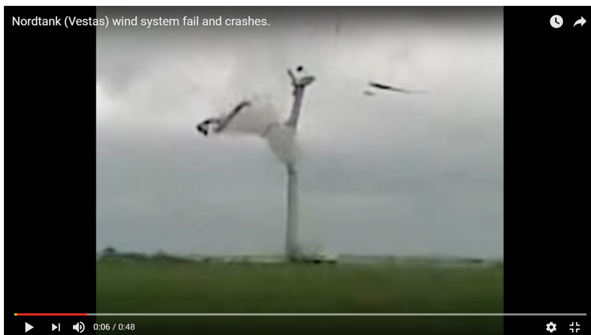
Figure 1.57. Frame of the video where a wind turbine is completely destroyed. Source: YouTube https://youtu.be/CqEccgR0q-o . Standard YouTube License.
