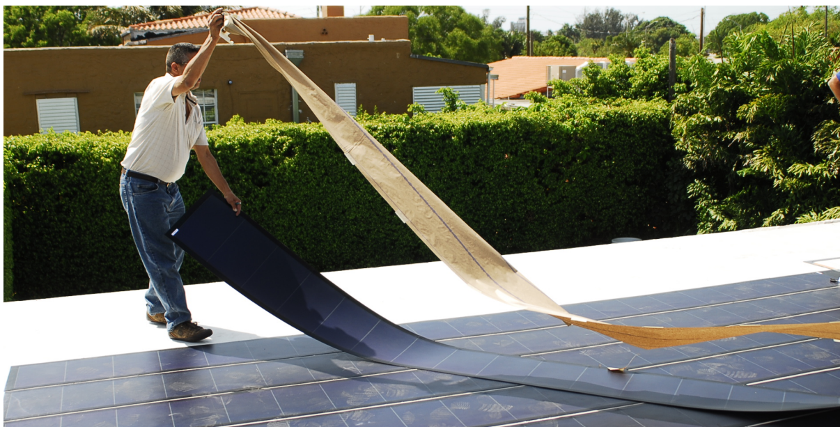
Figure 2.54. Thin film PV installation. Source: Fieldsken Ken Fields (CC BY-SA 3.0). http://bit.ly/21A2p1W .
