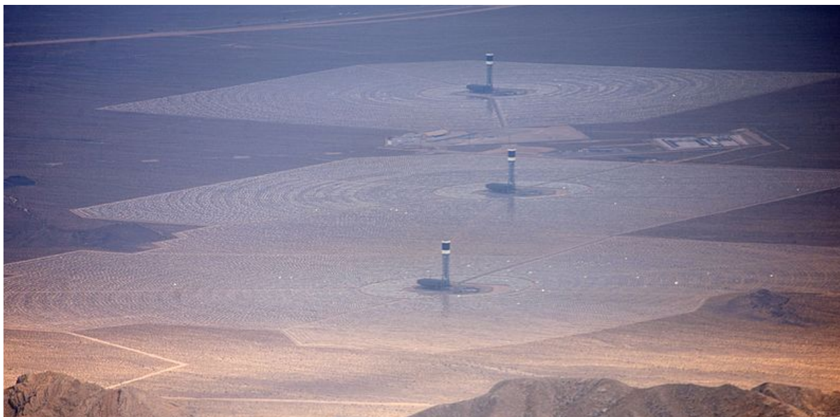
Figure 2.10. Ivanpah Solar Electric Generating System, at Mojave desert (California). Source: Craig Butz/CC BY-SA 4.0. http://bit.ly/2CWqPNF .
