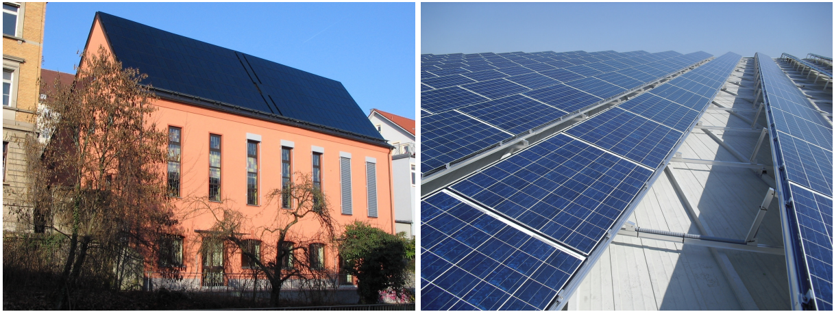
Figure 2.100. Examples of roof-top PV systems (left) using the inclination of the roof; (right) using a structure to establish a better tilt angle. Source: (left) Wikipedia http://bit.ly/2DgfpFH Free GNU License; (right) http://bit.ly/2CPua11 CC-BY-2.0
