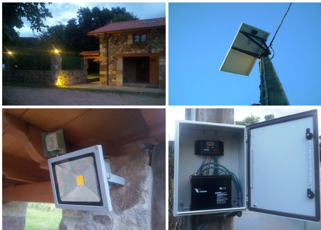
Figure 2.109. PV system images (from top to bottom and left to right): single-family home with the outdoor lighting system; detail of the installed PV module; 20W LED and PIR detector; charge controller and battery. Source: Instalación fotovoltaica aislada programable para alumbrado exterior con detector de presencia (David Lavín) . License: CC-BY-SA 3.0.
