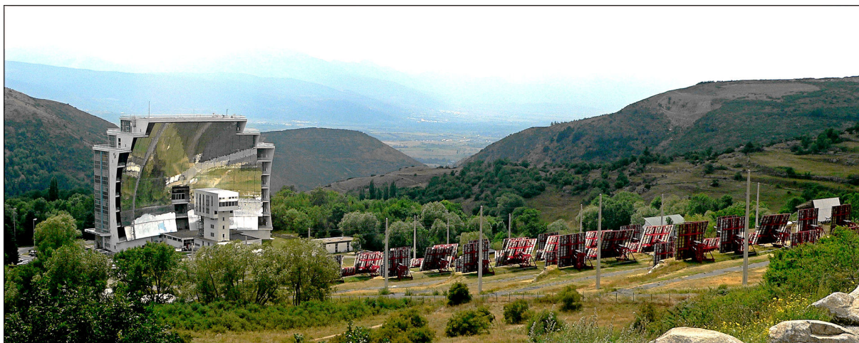
Figure 2.11. Solar thermal furnace installation in Odeillo (France). Source: http://bit.ly/2zewRXF . License: CC-BY-SA 3.0.
