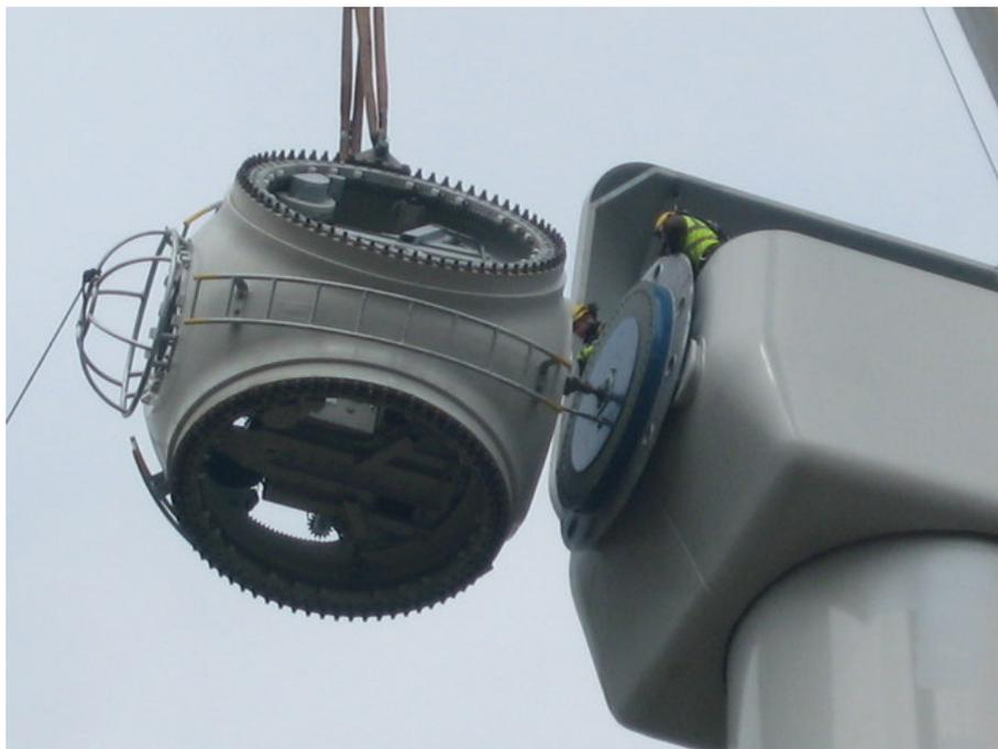
**Figure 3.36.** Wind turbine hub being connected to the nacelle. Source: Wikimedia. License: CC-BY-SA 2.0
