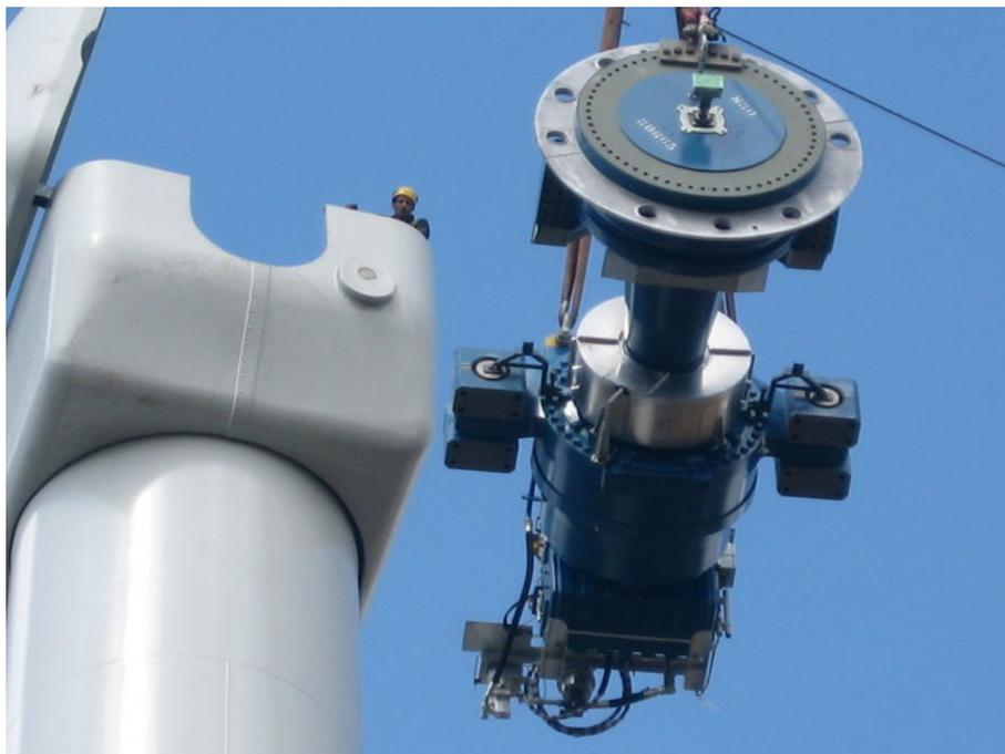
**Figure 3.40.** Gear box, rotor shaft and brake in a wind turbine. Source: Wikimedia. License: CC BY-SA 2.0. <http://bit.ly/2ERH8Mx>
