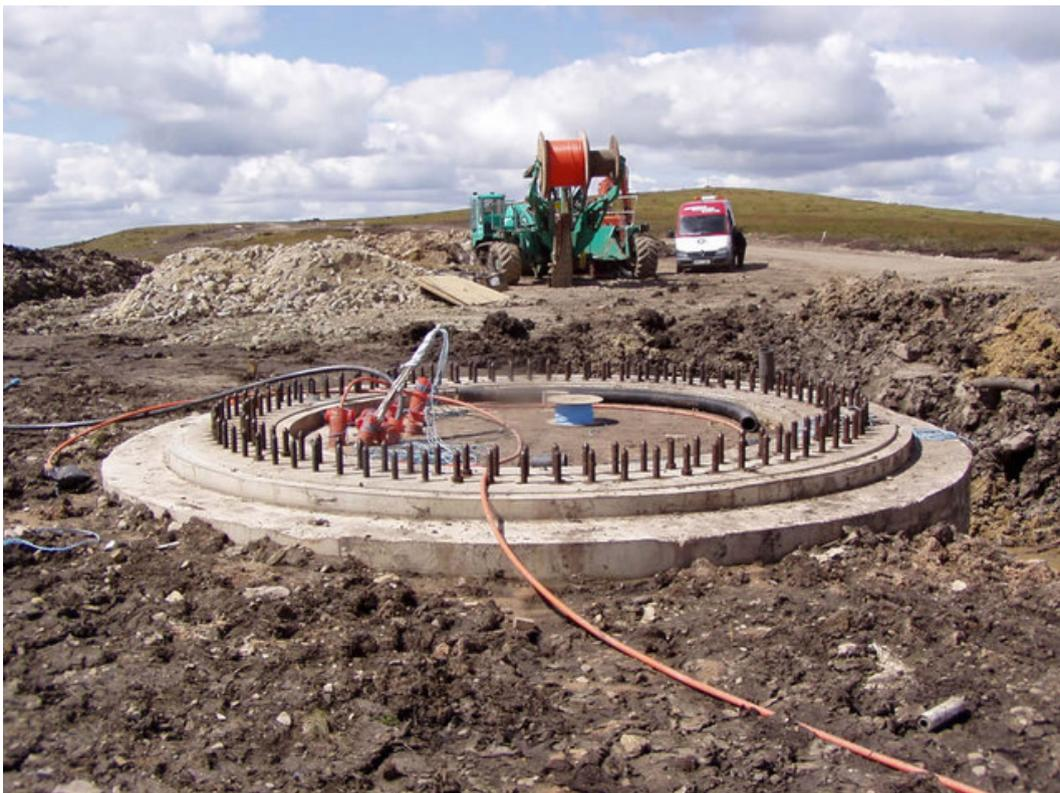
**Figure 3.30.** Foundations of an onshore wind turbine. Source: Wikimedia. License: CC BY-SA 2.0. <http://bit.ly/2mLQ6nZ>
