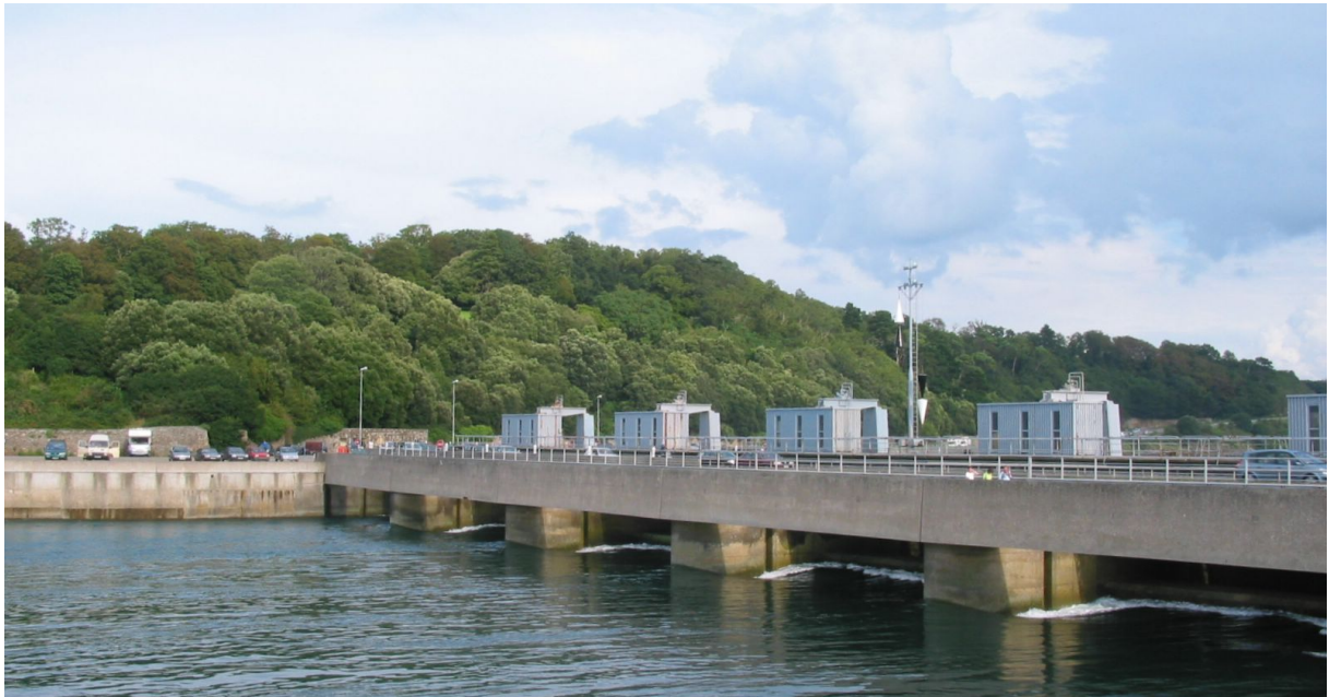
Figure 4.12. Rance river tidal power plant. Source: Wikimedia / Dani 7C3. License: CC BY-2.5 http://bit.ly/1GLZQ8g
