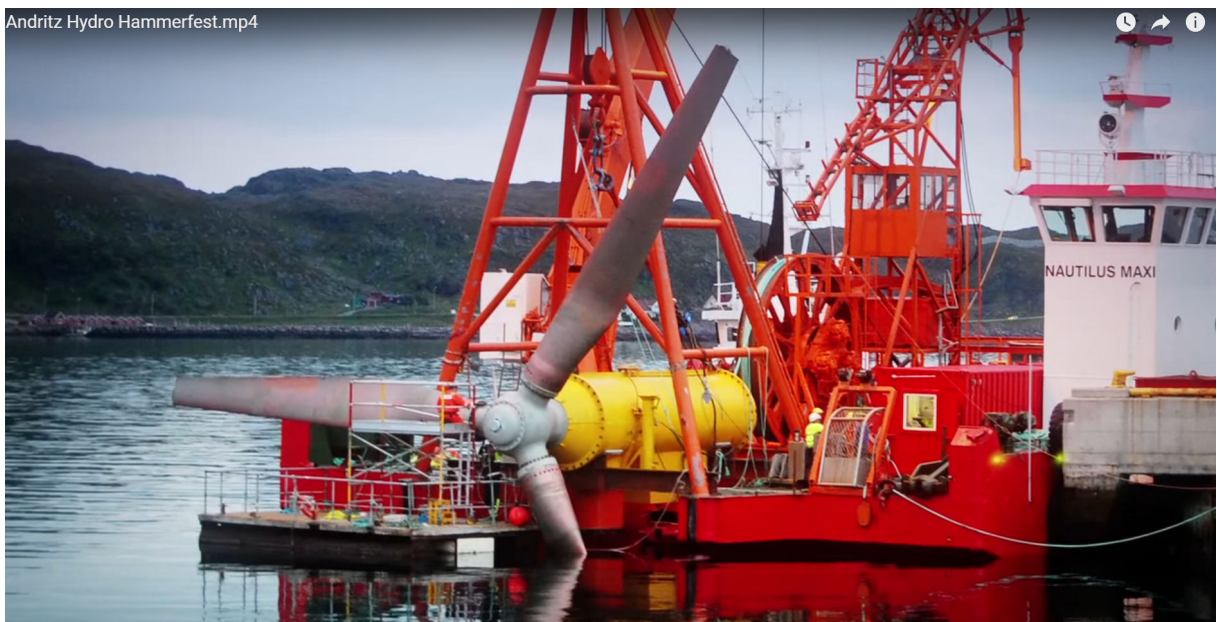
Figure 4.13. Installation of a Lanstrom turbine. Source: Andritz Hydro Hammerfest (hammerfeststrom). License: YouTube standard https://youtu.be/cHEXrBcdTck
