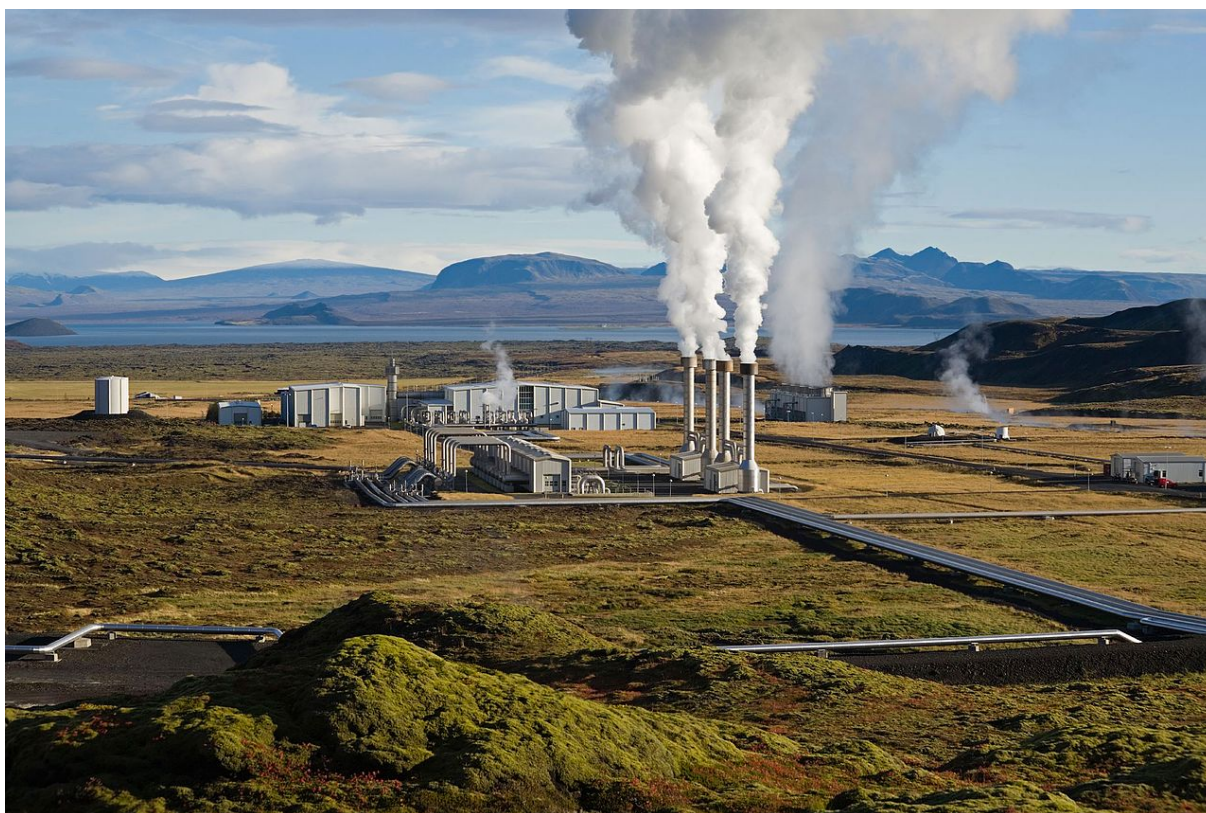
Figure 4.26. Geothermal power plant in Iceland. Source: Wikimedia / Gretar Ivarsson – Edited by Fir0002 - Gretar Ivarsson, geologist at Nesjavellir. The Nesjavellir Geothermal Power Plant in Pingvellir, Iceland. License: Public Domain http://bit.ly/2nJvk0v
