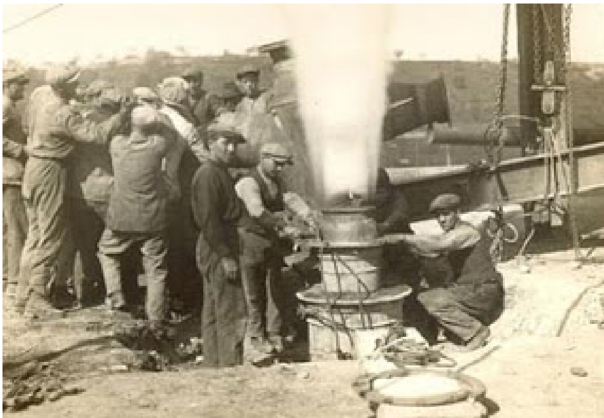
Figure 4.27. Larderello geothermal plant in 1913. Source: manodemandiocaambiente.blogspot.com.es http://bit.ly/2DH8dG8
