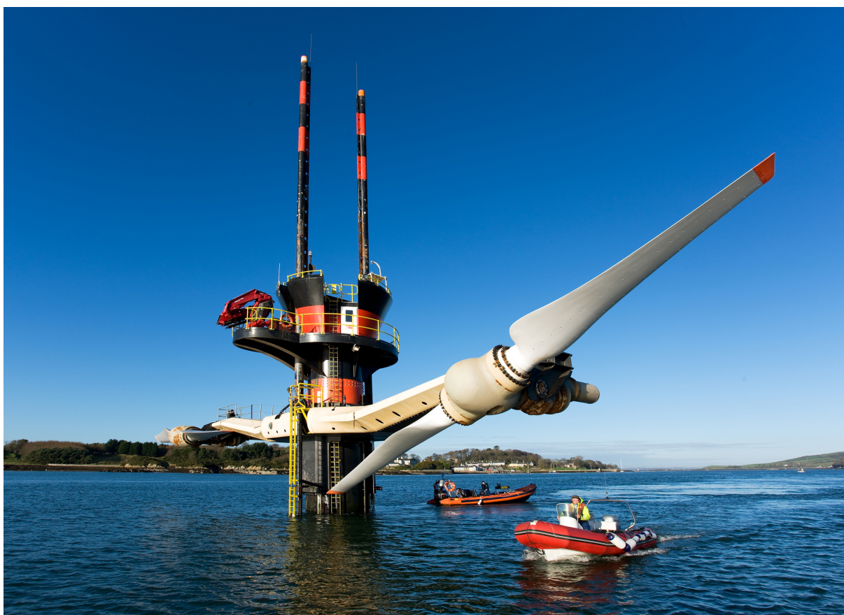
Figure 4.14. Seagen turbine. Source: Marine Current Turbines Limited http://bit.ly/2E8RVTr
