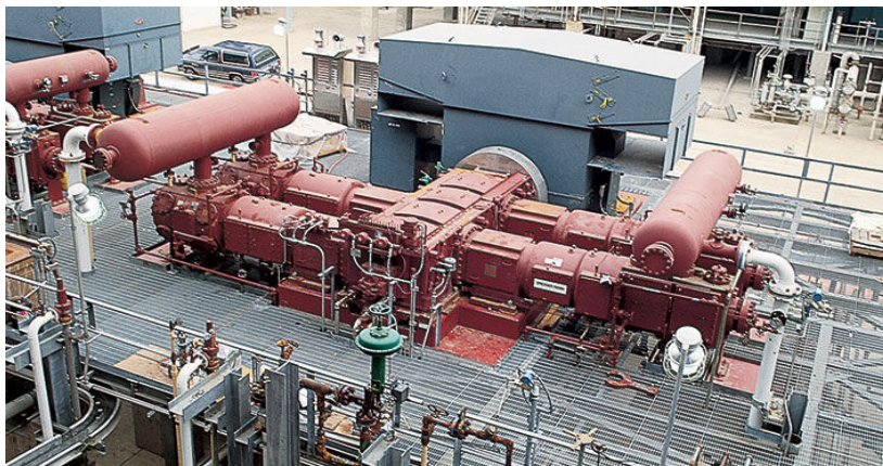
Process Gas Compressor Stationary Reciprocating Oil Injected.
