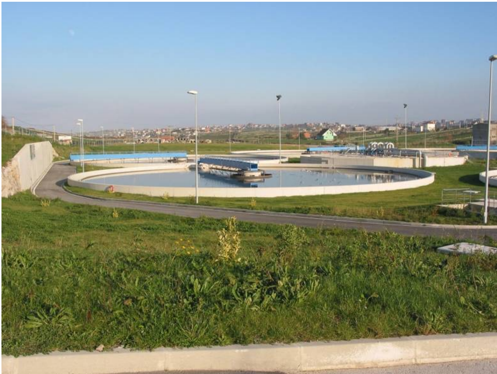
Secondary clarifier (WWTP of Santander)
