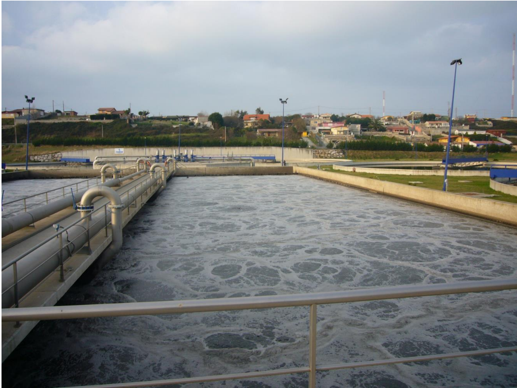
Biological reactor (aeration tank) (WWTP of Santander)
