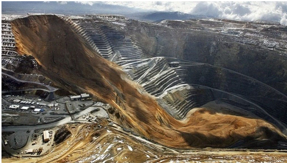
Bingham Canyon Mine (Utah, USA) landslide, 2013
