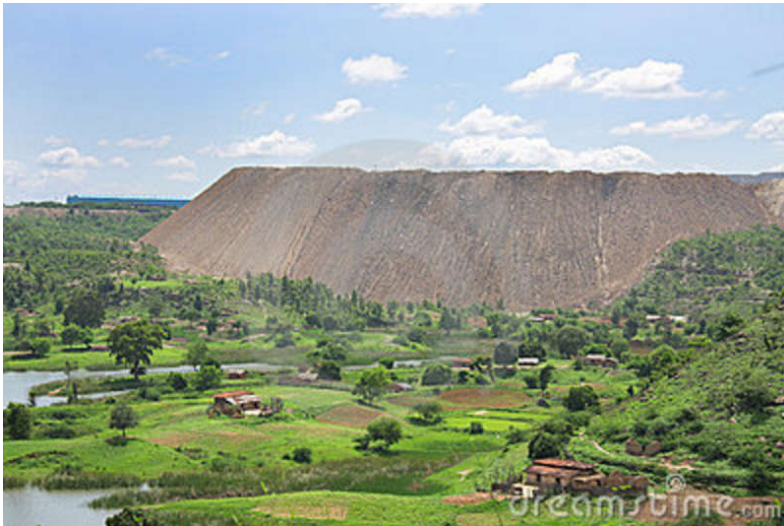
Waste rock dump
