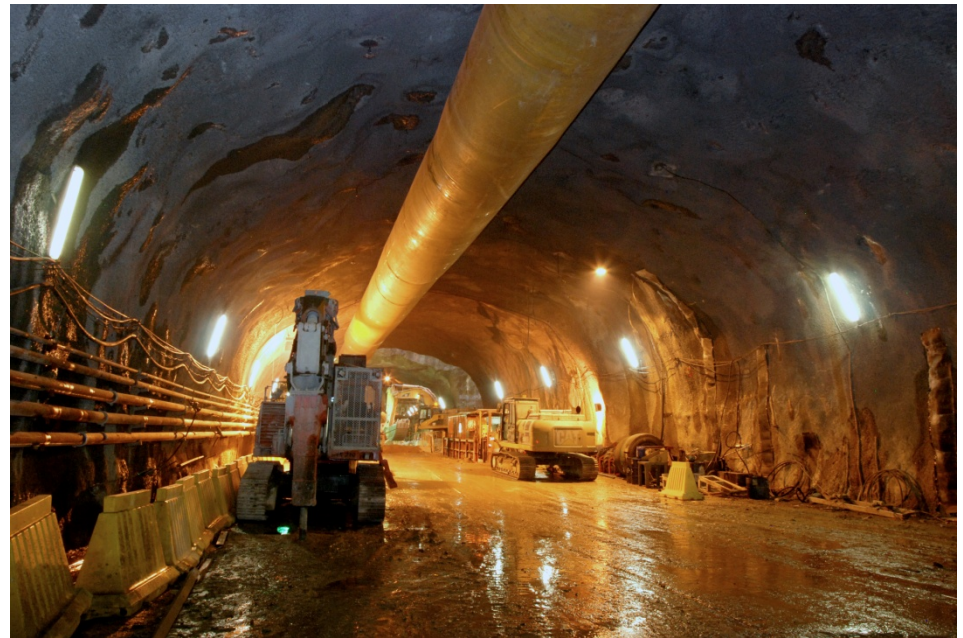
Example of duct system application
